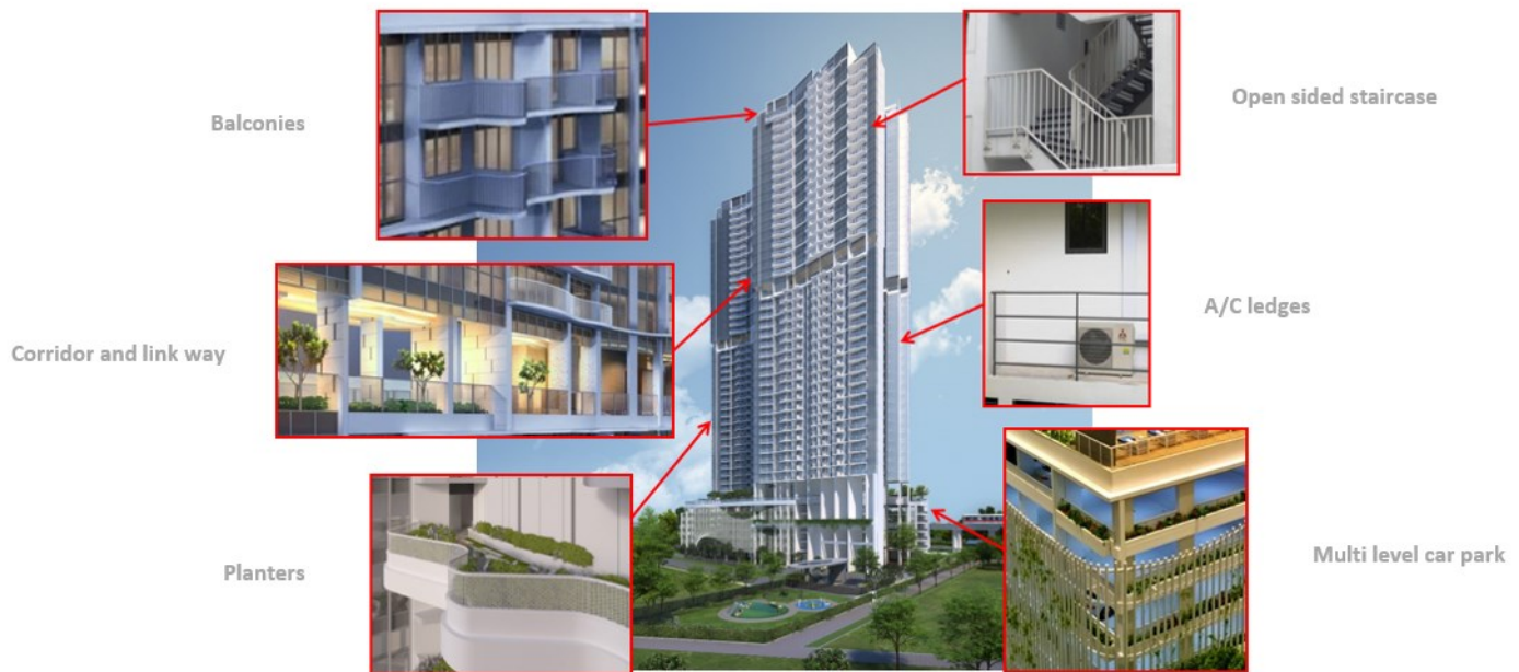
Areas affected by WDR. Image source: Fast Flow Systems Pte Ltd
